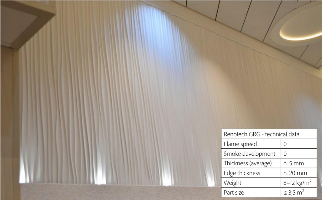
Renotech GRG is a non-combustible, glass fiber reinforced, alfa gypsum based, moulded product. GRG mouldings are light-weight, durable, easy to handle and install.
