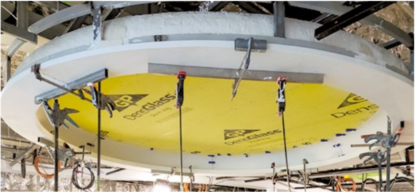
Renotech DGG is fastened to solid steel structure with adhesive and screw's.
