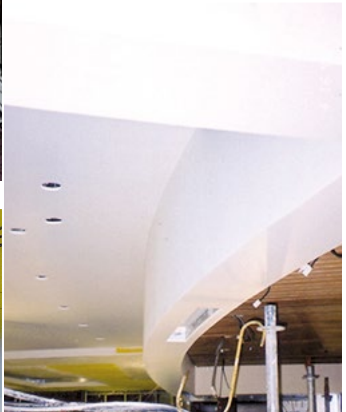
Renotech DGG can be bent to shape (see Properties for bending radius, p. 4).
