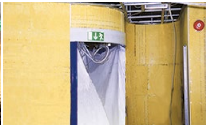
Renotech DGG can be bent to shape (see Properties for bending radius, p. 4).
