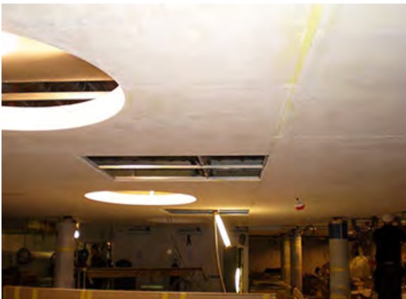
CA-120 adhesive gypsum plaster coated DGG sheet (point 3)
