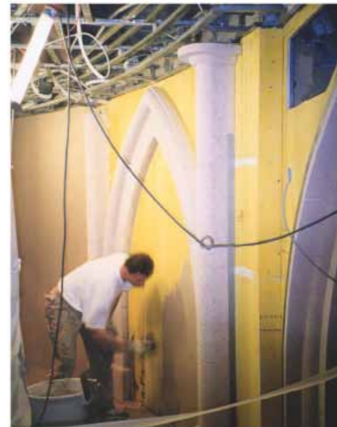
As substrate for Renotech Stonemix 54 trowel applied surface
